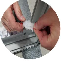
Connect the three LED-DB-PWRSUPLY-2-CL-2500 (x3) to each other and feed until it exits the grommet hole at the top of the right side of the frame.
