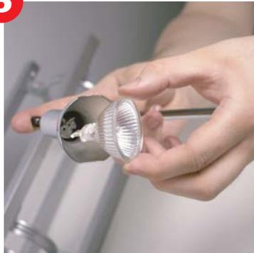
To replace light bulb, hold bulb from sides with fingertips. Line up the 2 metal prongs on the bulb with holes in socket and firmly push into place.
